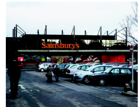
This modern supermarket contributes nothing to the special interest of the Conservation Area
